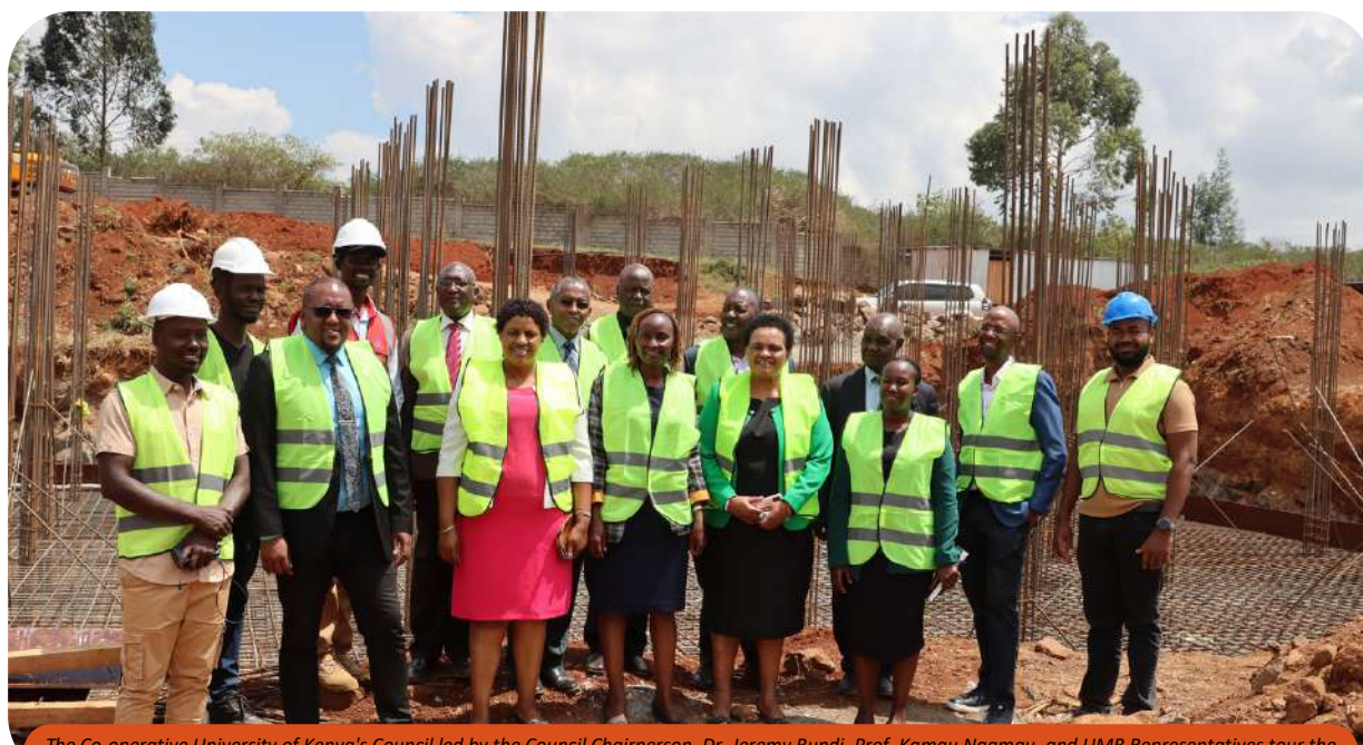
The Co-operative University of Kenya's Council led by the Council Chairperson, Dr. Jeremy Bundi, Prof. Kamau Ngamau, and UMB Representatives tour the 2,500-capacity student hostels being constructed under the Affordable Housing Programme on 28th November 2025.
